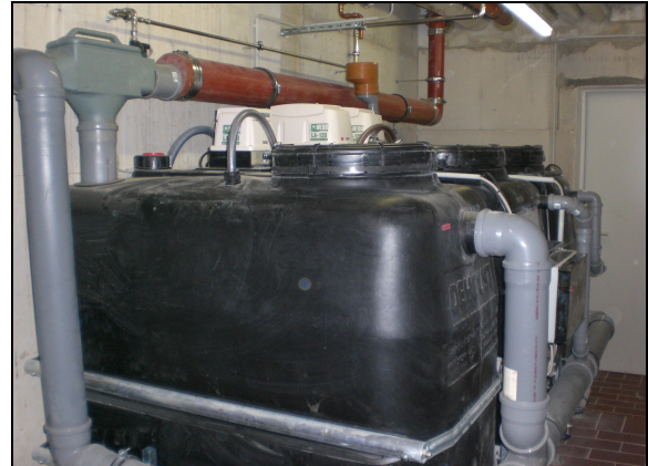
The space-saving GEP grey water unit in the Krankenhaus Nettetal takes up a mere 4.5 m 2 .
