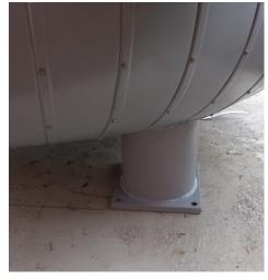
Placing the vessel on the foundation and marking of the drill holes.
