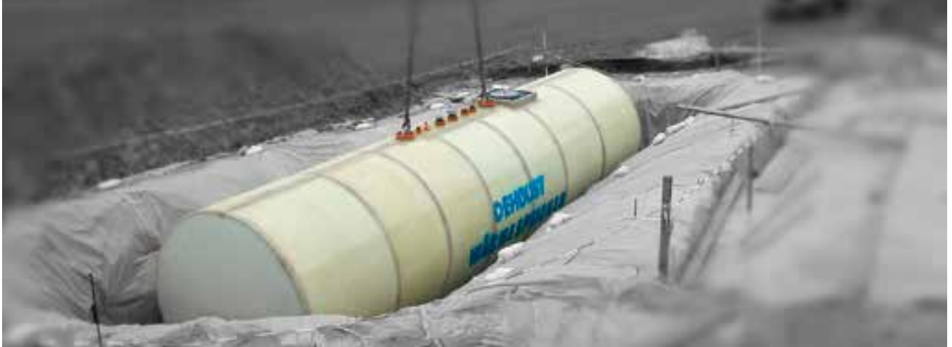
Horizontal underground heat storage tanks operating pressure 6 bar
